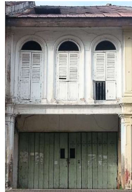
The facade of the Arlene Terrace before restoration work began.
