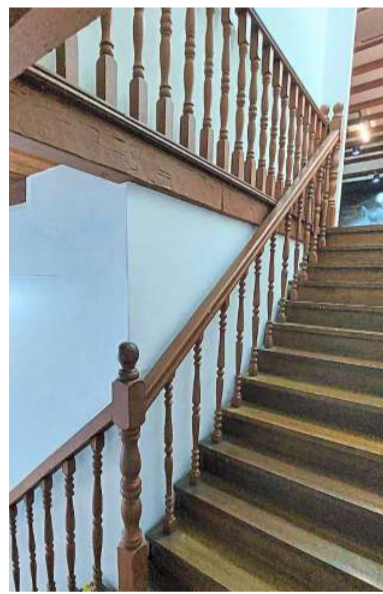
(Left) The original cengal staircase and balusters at Arlene Terrace.
