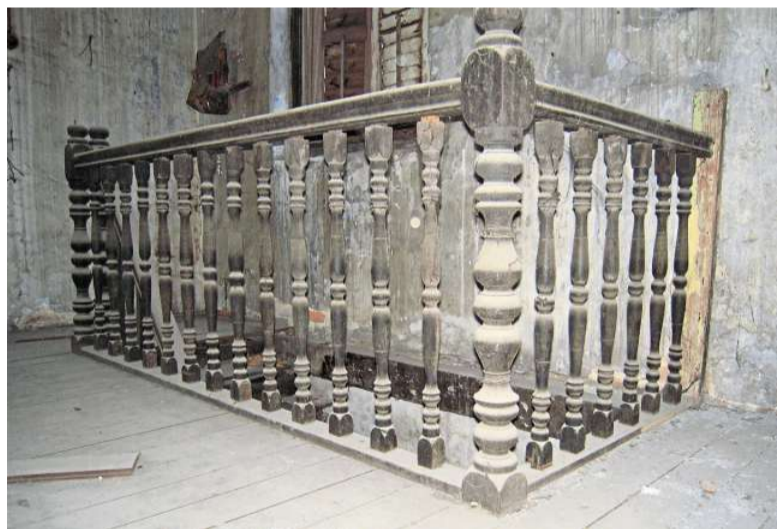
(Left) The original cengal staircase and balusters at Arlene Terrace.
