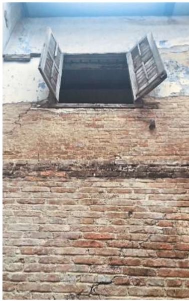
The courtyard with its British-era clay bricks before the restoration.
