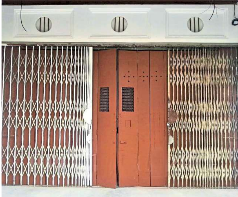
The Anderson Gates which were salvaged from another colonial shophouse and restored at the Arlene Terrace.
